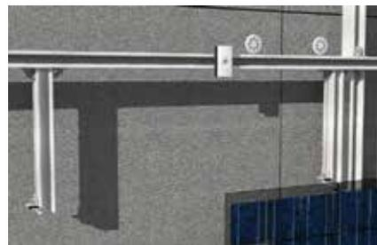
Detail: vertical profile VP 50 connection
