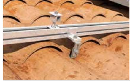
Detail: fixing of profile Solar on hook GTU
