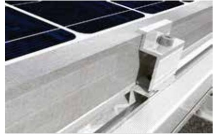
Detail: fastening of PV module
