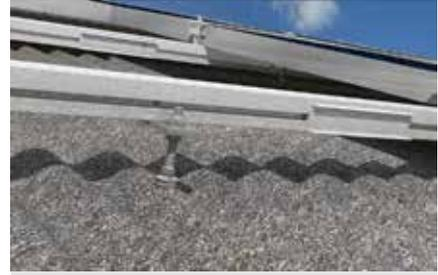
Detail: Stud screw STSI with bracket SSP
