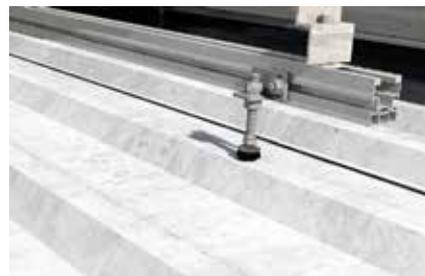
Detail: Joint bracket MW SU
