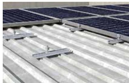
Installation on industrial roof with Solar-flat P 400
